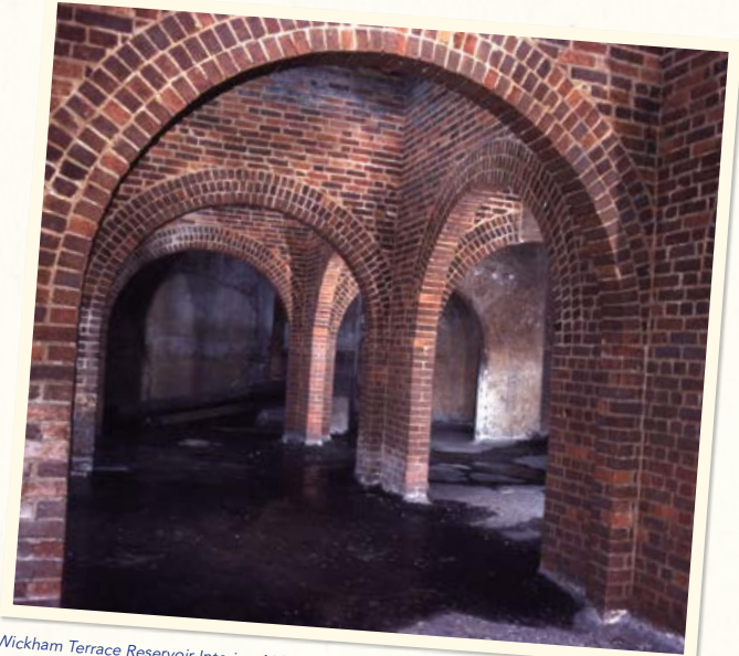
Wickham Terrace Reservoir-Interior, 1983, Brisbane City Council, BCC-S35-939654
