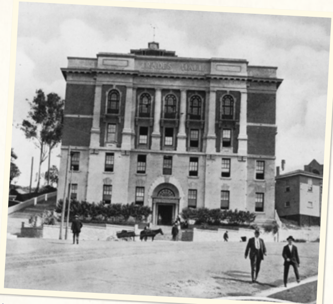
View of Trades Hall Building in Brisbane, ca. 1928, State Library of Queensland, Negative Number 71110
