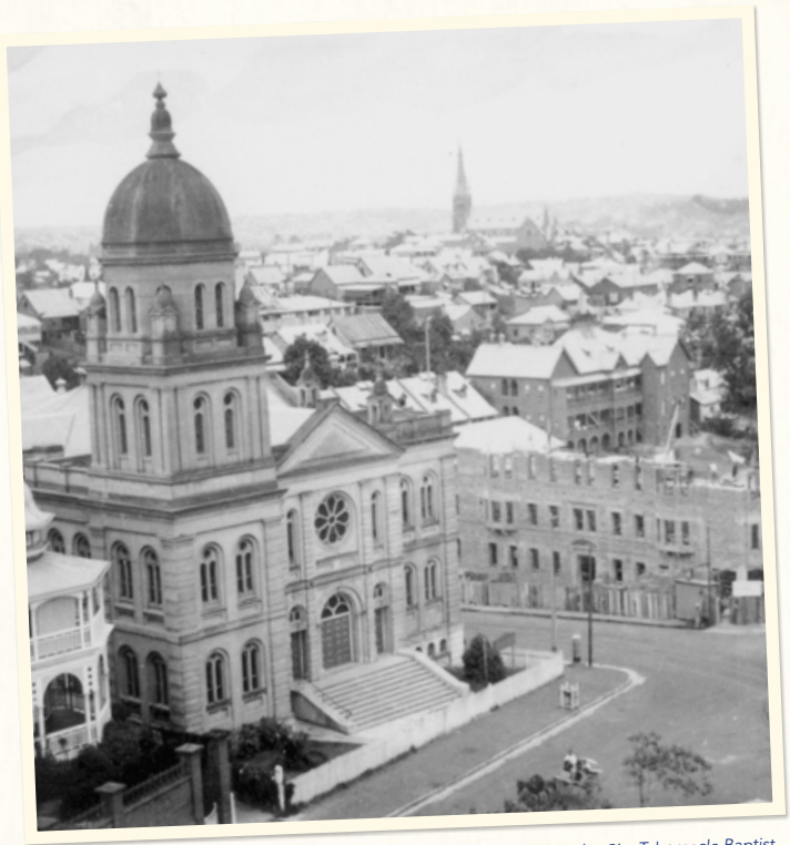
Corner of Wickham Terrace and Upper Edward Street, Brisbane, including the City Tabernacle Baptist Church, 1923, State Library of Queensland, Negative Number 182797
