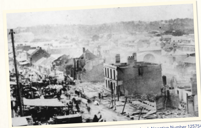
Great Fire in Queen Street, Brisbane, 1864, State Library of Queensland, Negative Number 125754
