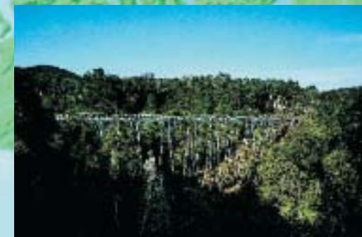
Percy Burn Viaduct, Tuatapere Hump Ridge Track
